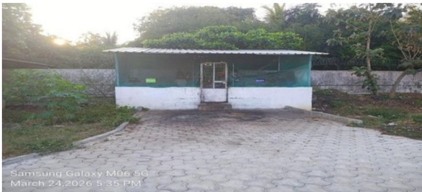
Pic: Covered and Fly Proof Garbage Yard
