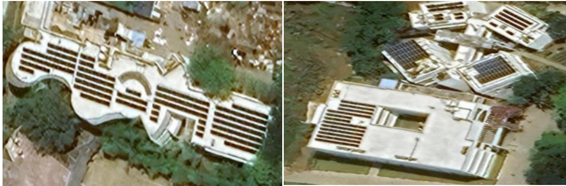
Pic : 147 KW power Solar Panels
