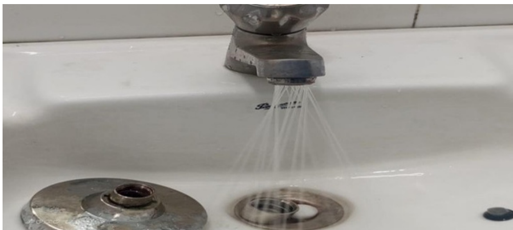
Pic: Flow Conservators for Washbasin Taps
