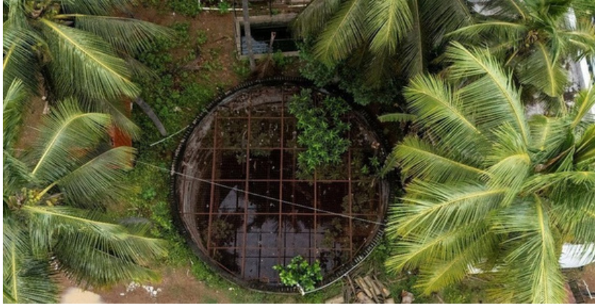
Storage Well 2 – constructed inside the campus for water storage
