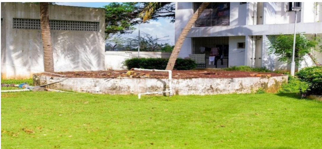
Storage Well 1 – constructed inside the campus for water storage
