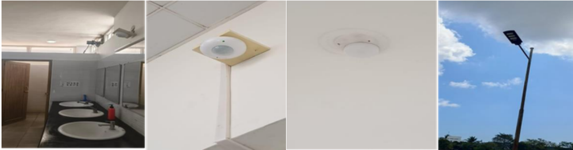
Pic: Motion sensor-based lighting
