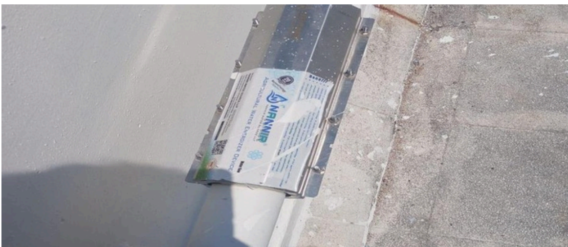
Pic: Descaling of Water pipelines using Ultrasound Technology
